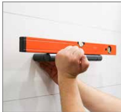
Simple alignment of the handle. A single strike of the handle marks the second drill hole.
