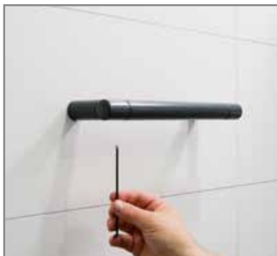
Screw in the set screws and tighten.
