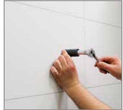
Mount the fitting on the wall.
